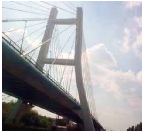
Otopeni Bridge - Romania
