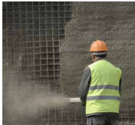
Tunnel T-48 - India
