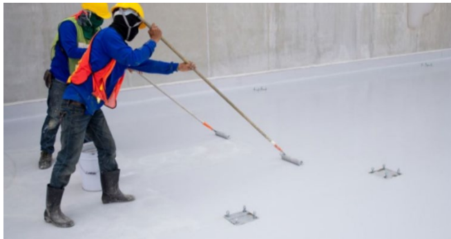
Application of Aquathane E400
