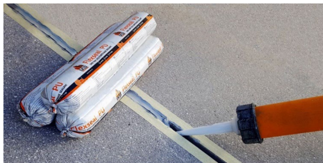
Application of Flexseal PU425/440 in joints
