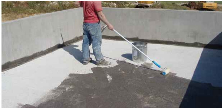
Application of Aquathane E400 diluted with water as a primer
