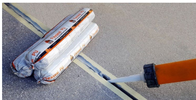
Application of Flexseal PU425/440 in joints
