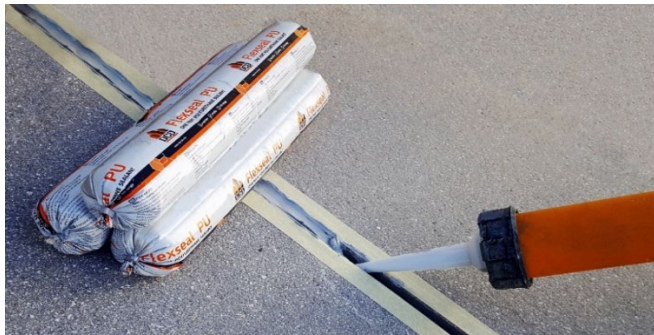
Application of Flexseal PU425/440 in joints
