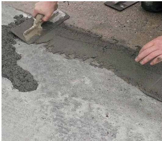
Repair of surface imperfections using cementitious repair mortar
