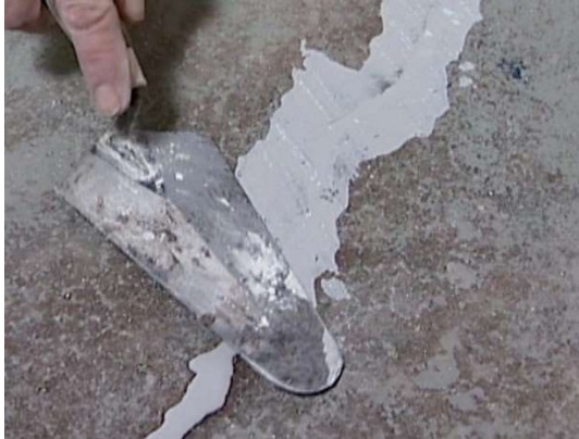
Repair of cracks using Flexseal PU245 or PU440
