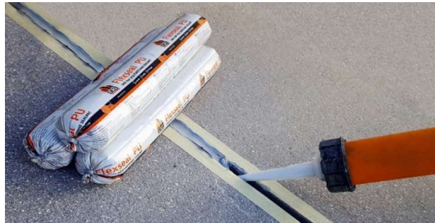
Application of Flexseal PU425/440 in joints
