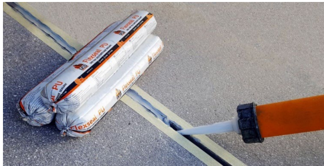
Application of Flexseal PU425/440 in joints
