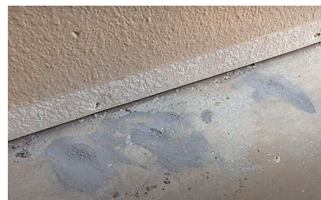
Repair of surface imperfections using cementitious repair mortar
