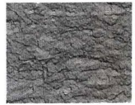
CSP 6 (medium scarification)
