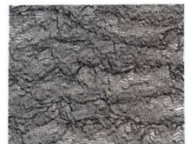
CSP 9 (heavy scarification)
