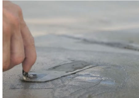
Repair of pinholes and surface defects
