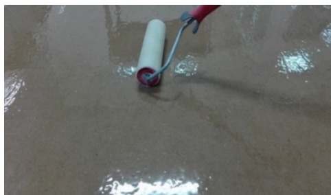
Application of Gripdeck Primecoat U
