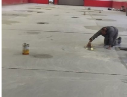
Repair of pinholes and surface defects
