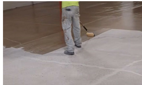
Application of Gripdeck Primecoat U
