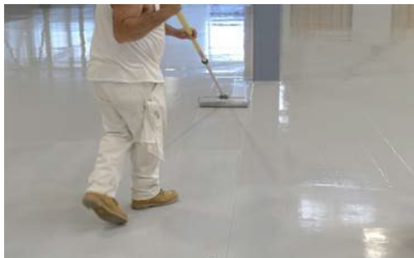
Application of Gripdeck Wearcoat TE using Roller
