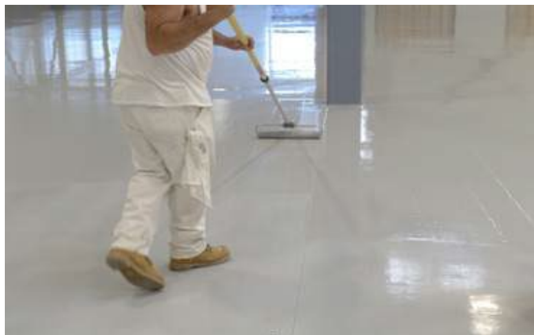
Application of Gripdeck Wearcoat TE using Roller
