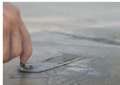
Repair of pinholes and surface defects
