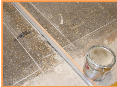
Masking tape & saw cutting around the floor
