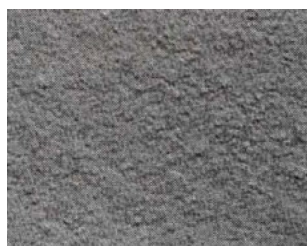
CSP 3 (light shot-blast)
