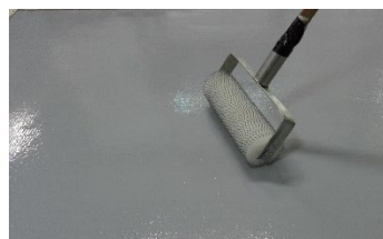
Spiking of Strongcoat Conductive Topcoat F
