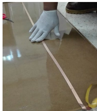
Placement of copper tape
