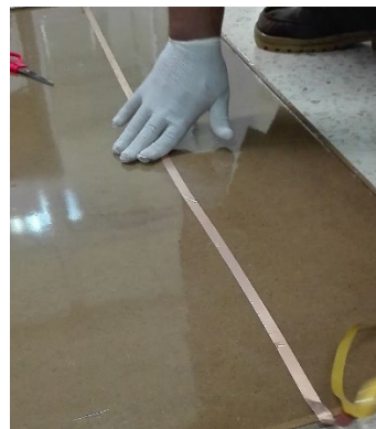
Placement of copper tape
