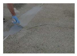
Note: If the surface is contaminated by oil or grease, it is recommended to treat such areas with hot compressed air.
