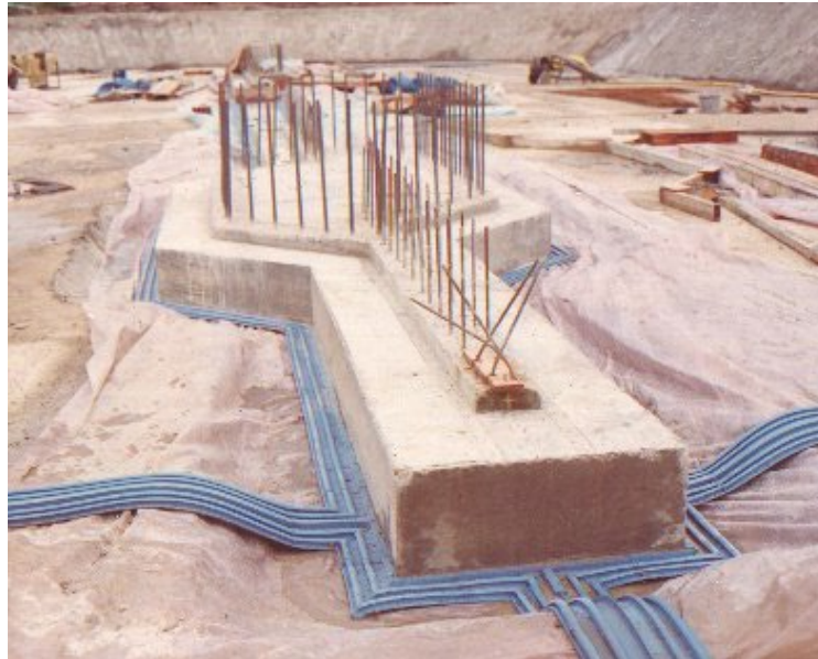
Externally fixed PVC waterstop
