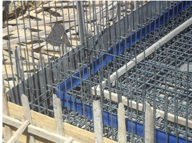
Properly fixed PVC waterstop
