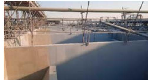
**Quickmast 341** enabled effective filling of blowholes and surface imperfections, creating a smooth and uniform substrate essential for achieving optimal adhesion and long-term coating performance.
