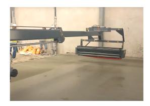
After the concrete has been floated, and light foot traffic would leave an imprint of about 3 - 6 mm (a guarter of an inch), it was ready to receive the dry shake hardener TIBMIX. For large floor constructions, TIBMIX was spread and trowelled satisfactorily in one stage by mechanical spreaders.
